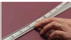
Lay Light In Channel
