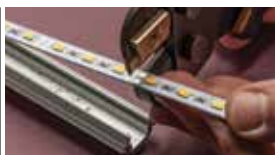
Measure & Cut Thin Strip Where Marked
