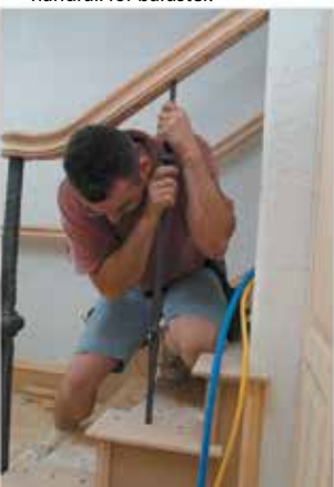
7. Install baluster into epoxy filled holes and press in for tight fit.
