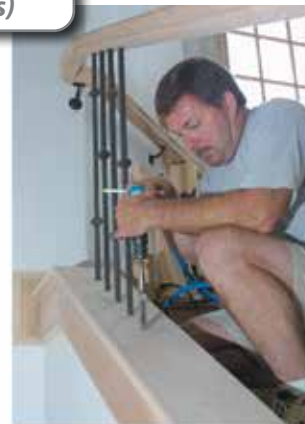
4. Square off bottom hole with air hammer/chisel and mortising bit without the drill inside. (For installation of square balusters without needing shoes)
