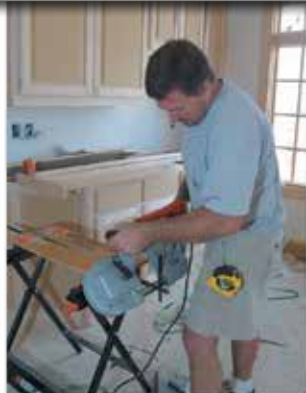
2. Cut baluster to length.
